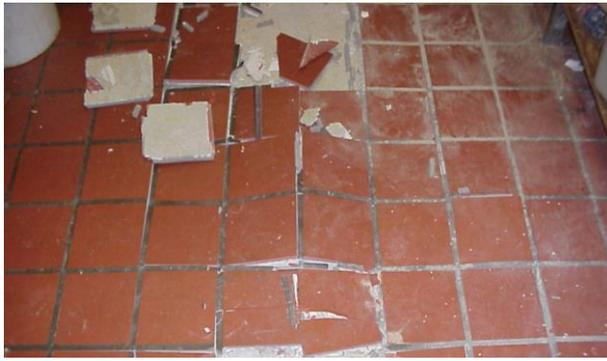
Fig.6. Popped Tiles on Corner Slab
