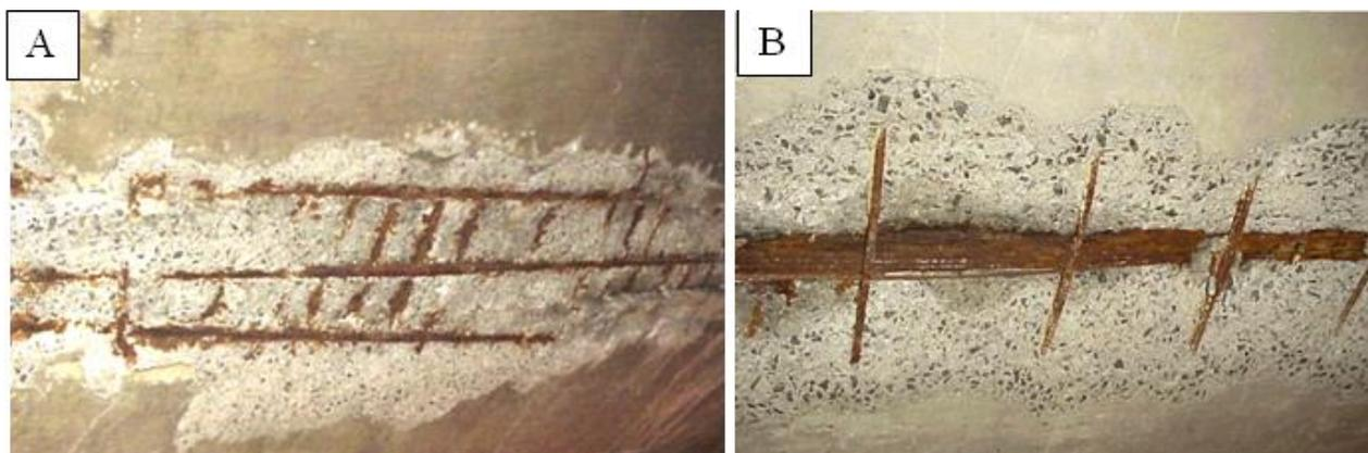
Fig. 8. Deteriorated Concrete and Rusted Reinforcement at the Bottom of Ramp Slabs:
