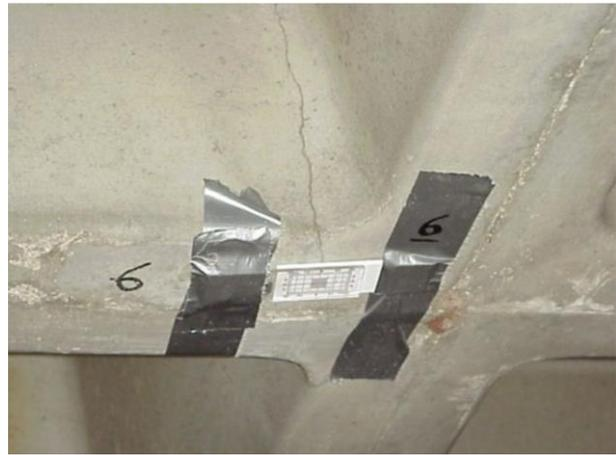
Fig.7. Monitor on the Crack on the Waffle Slab Rib
