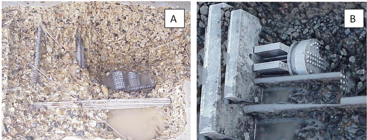
Fig. 9. Open Reinforcing (A) and Anchor (B) after Concrete Chipping
