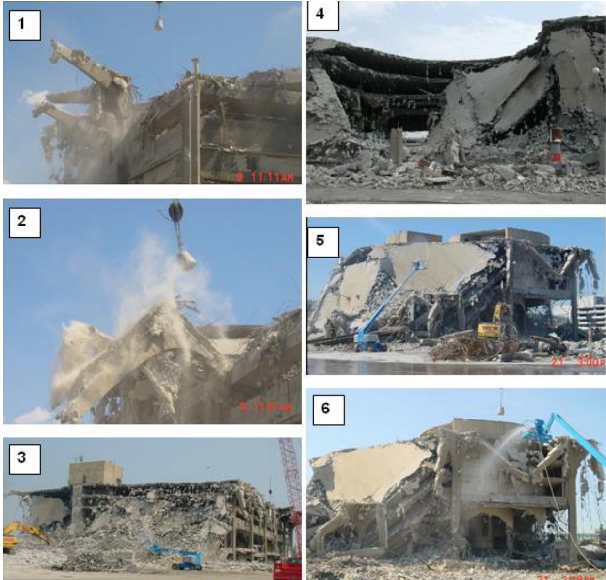
Fig. 11. Phases of Demolition (sequence follows the numbers)
